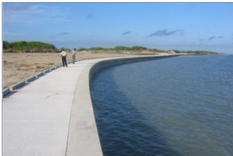
Figure 36. Example of Concrete Panel Bulkhead with Sidewalk
