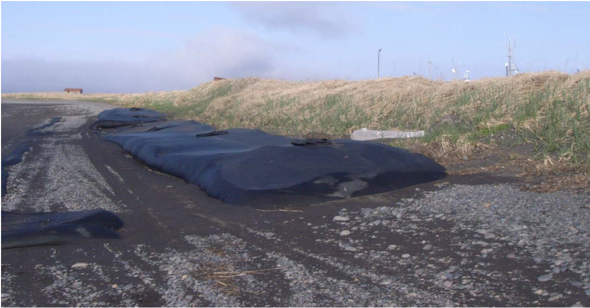
Figure 24. Geotube Containment Structure
